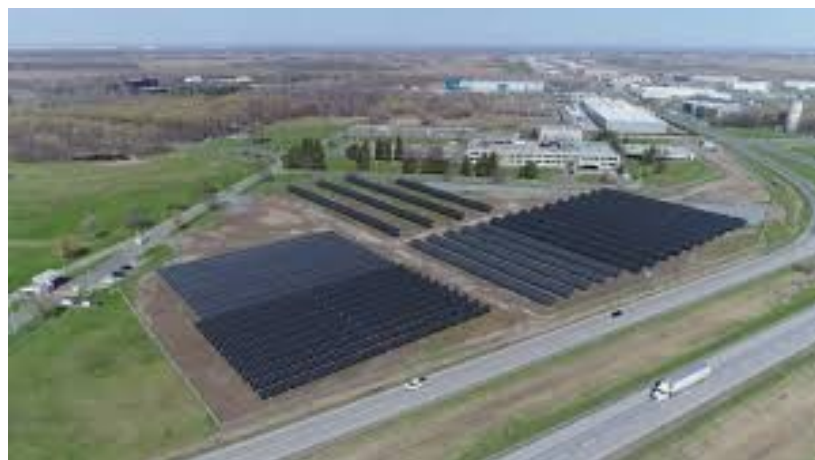
Centrale solaire Robert-A-Boyd – 2021 – Hydro-Québec
